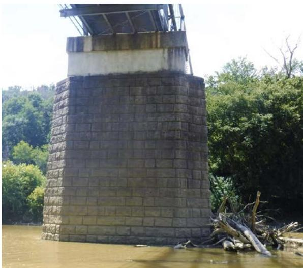
Figure 2: Old Clays Ferry Bridge over Kentucky River – Concrete Encased Pier with Rock Imprint
